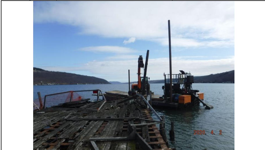
7.) Looking Northwest. The existing wood pile located at the Northeast corner of the existing Pier almost removed.
