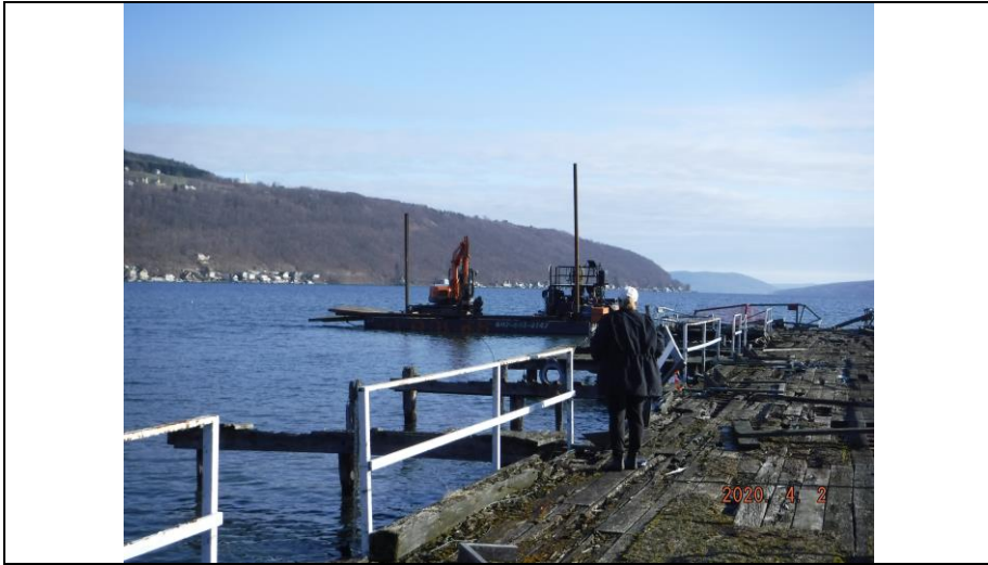
1.) Looking North. A view of the barge moving into position to install the Test Pile at the Primary Location off the Northwest corner of the existing Pier.
