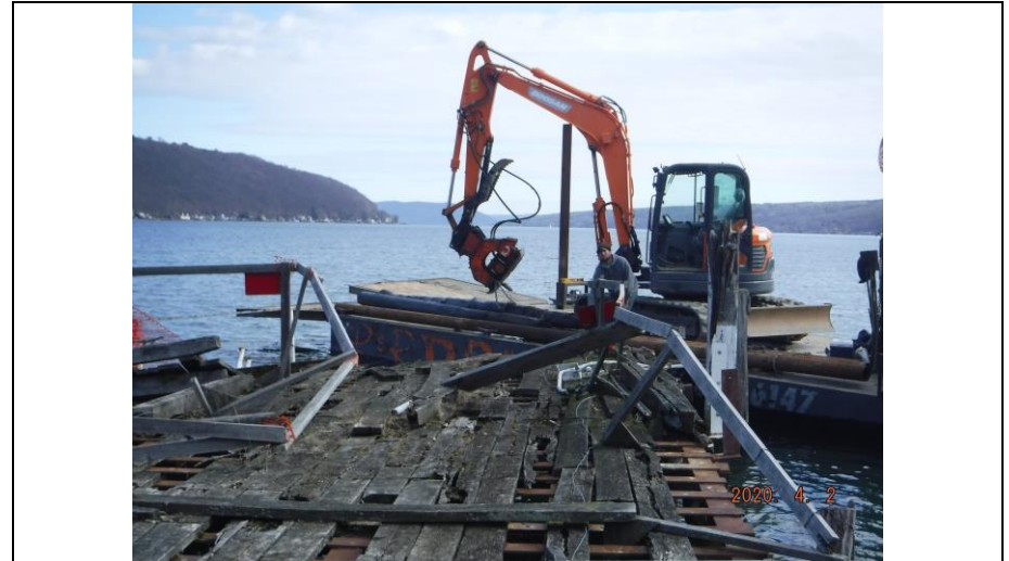
8.) Looking Northwest. The existing wood pile removed from the existing Pier being placed on the barge.
