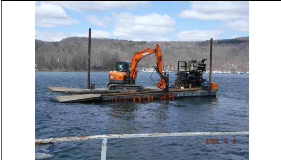
11.) Looking West. The excavator removing the Test Pile at the Primary Location following satisfactory results from the "Pipe Freeze" test.
