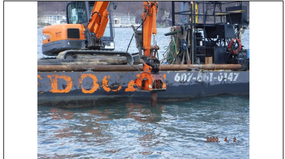
10.) Looking Northwest. A closeup view of the barge adjacent to the previously installed Test Pile at the Primary Location performing the test to evaluate "Pipe Freeze".
