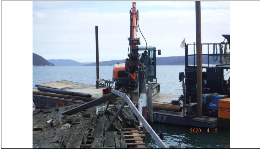
5.) Looking Northeast. A view of the barge in position off of the Northeast corner of the existing Pier in the process of removing an existing wood pile to determine embedment of pile.
