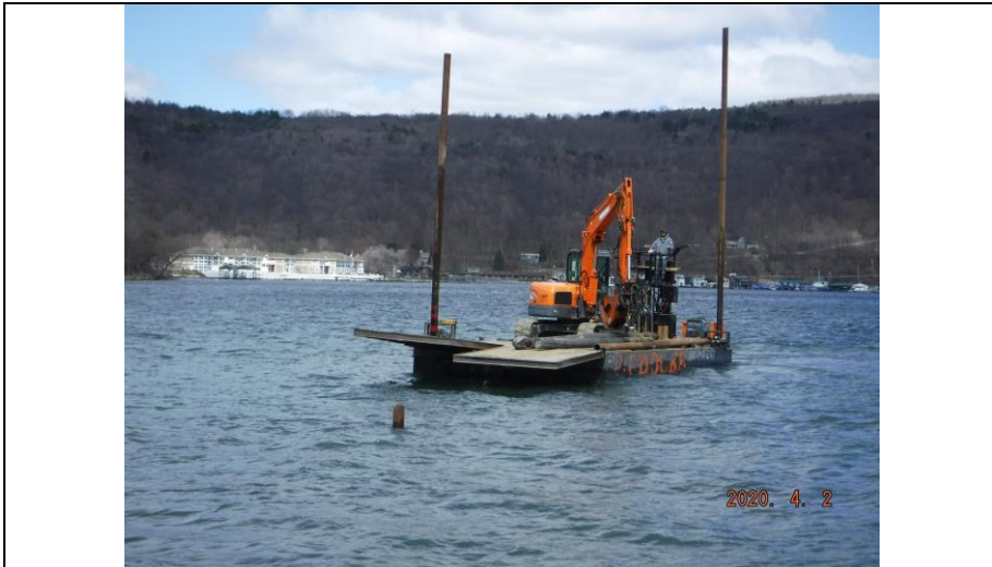
9.) Looking Northwest. A view of the barge approaching the previously installed Test Pile at the Primary Location to perform a test to evaluate "Pipe Freeze".
