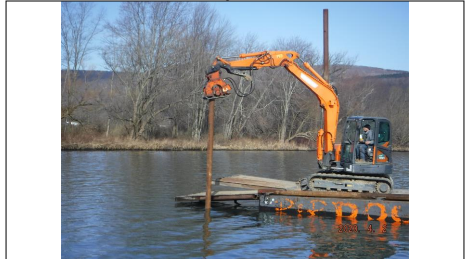
4.) Looking West. Another view of the Test Pile at the Secondary Location being driven by the hydraulic vibratory attachment on the DX85R Doosan Excavator w/thumb.
