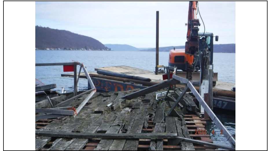
6.) Looking Northwest. A closeup view of the existing wood pile removal. Note the previously removed wood pile lying on the barge.
