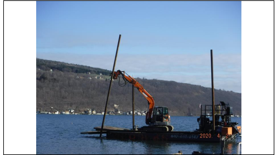
2.) Looking Northwest. A view of the Test Pile at the Primary Location being positioned at the proposed location approximately 42.3' away from the Northwest corner of the existing Pier.
