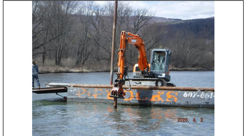
12.) Looking West. A closeup view of the barge adjacent to the previously installed Test Pile at the Secondary Location performing the test to evaluate "Pipe Freeze".
