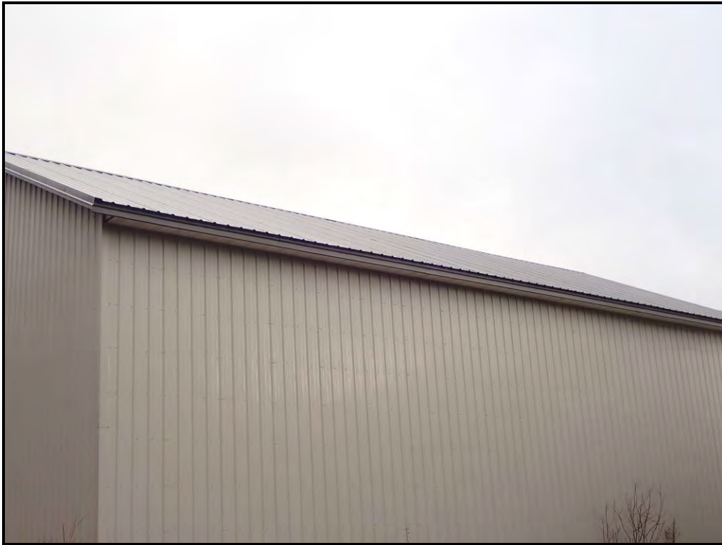
Non-Suspect Metal Roof / Walls
