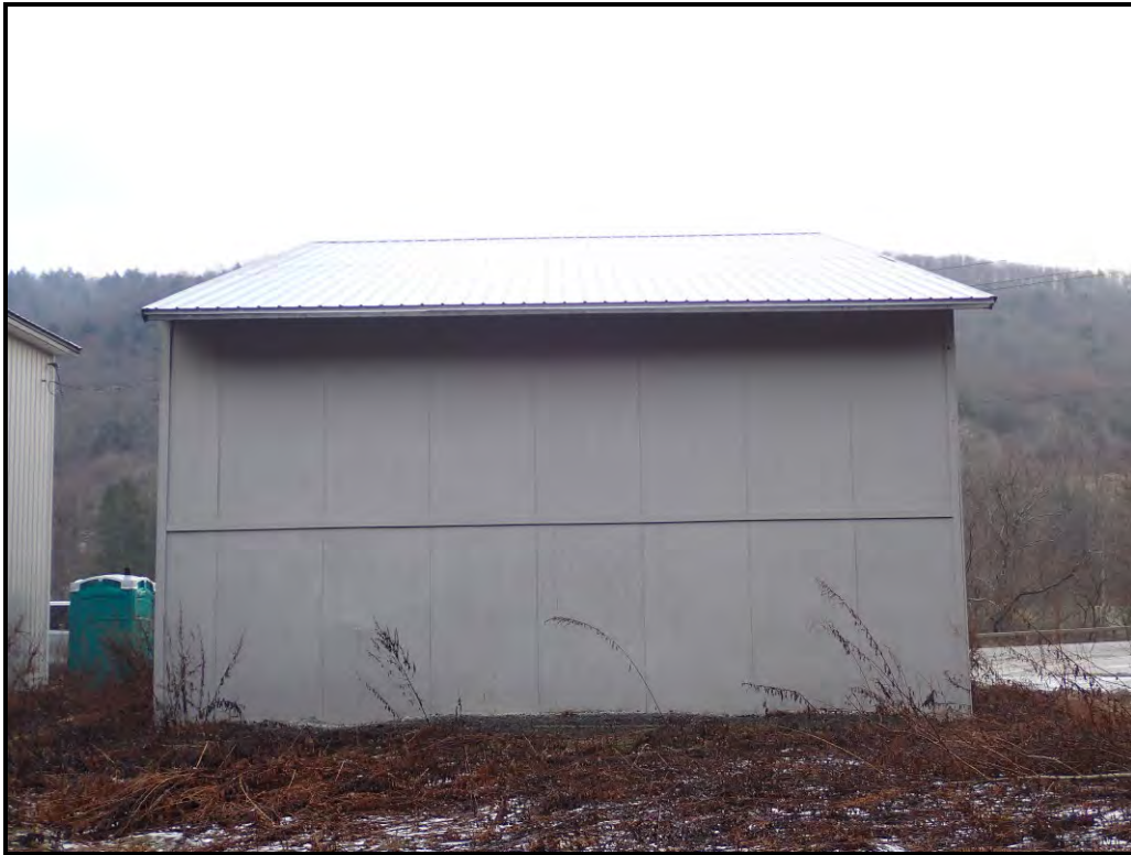
Non-Suspect Metal Roof / Wood Panel Walls
