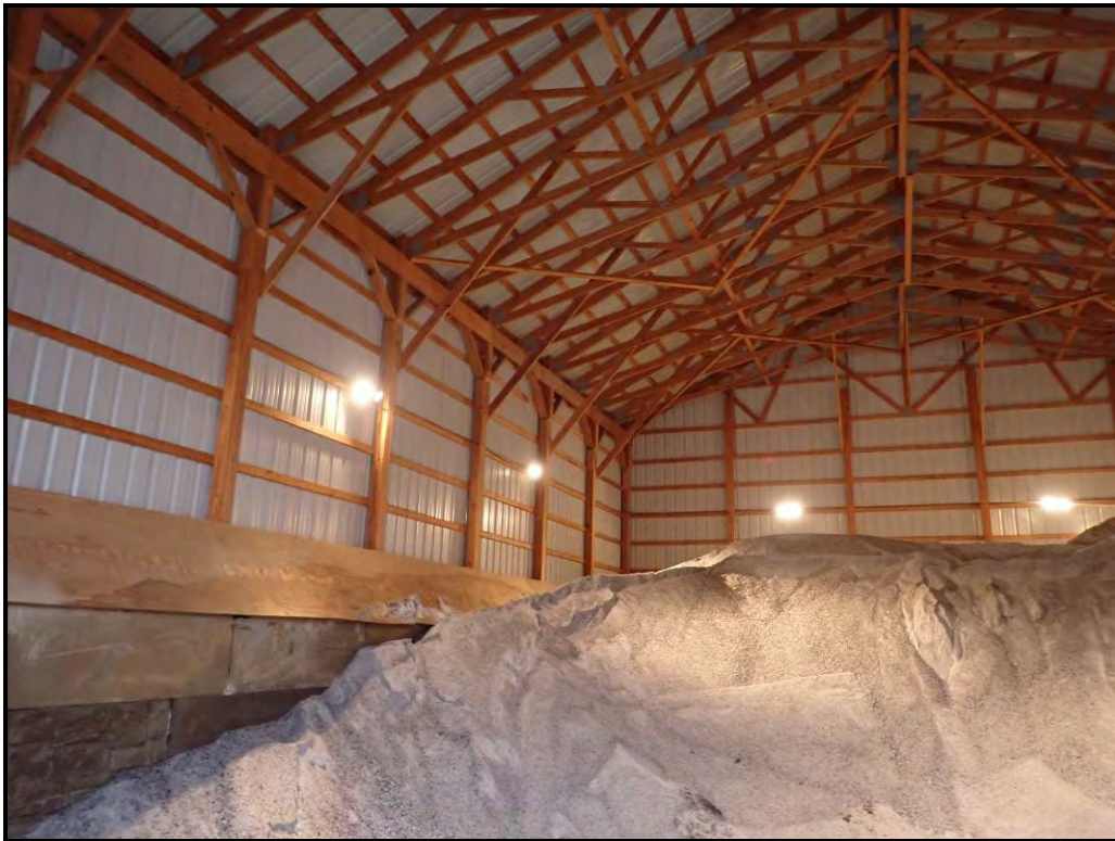
Non-Suspect Wood Structural / Framing Components
