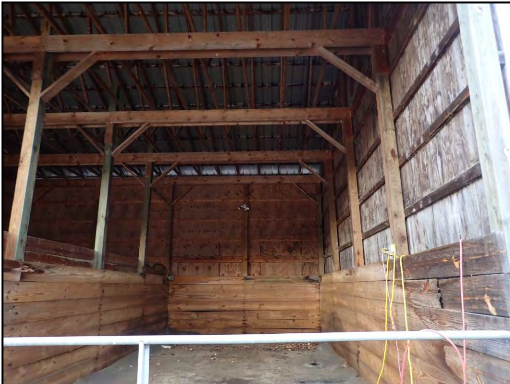
Non-Suspect Wood Structural / Framing Components
