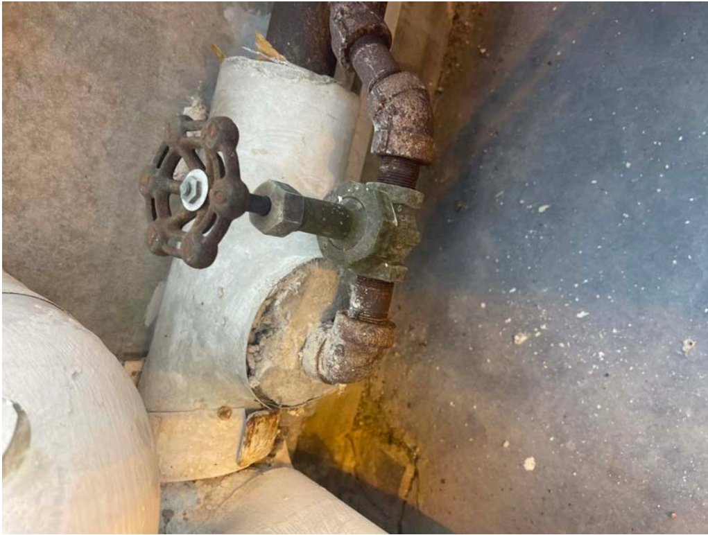
Photo #1: HAN400- Mudded Elbow Joints
