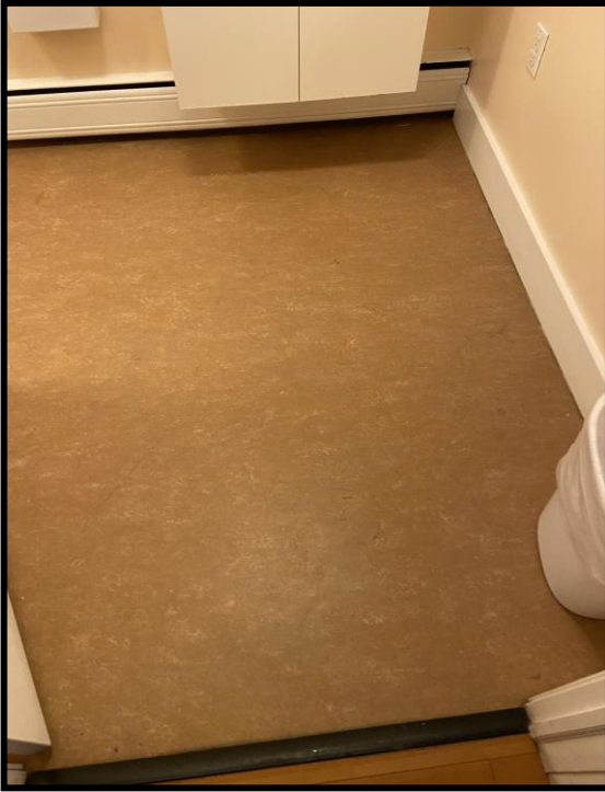
1 st FLOOR BATHROOM ADJ. FOYER, LINOLEUM FLOORING NOT SAMPLED AT THIS TIME, ASSUME 9" FLOOR TILE/MASTIC IS PRESENT BELOW.
