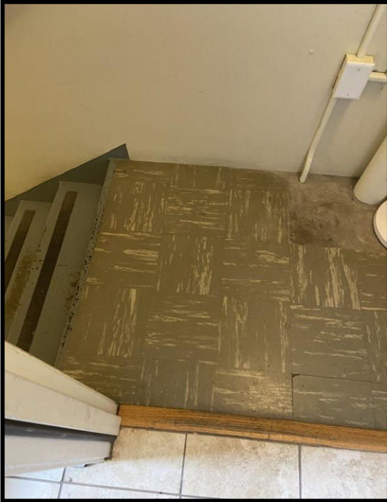
ACM 9" x 9" FLOOR TILE AND ASSOCIATED BLACK MASTIC IN STAIRWELL TO BASEMENT
