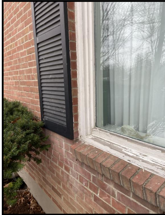
ACM EXTERIOR WINDOW CAULK (FRAME TO BRICK)
