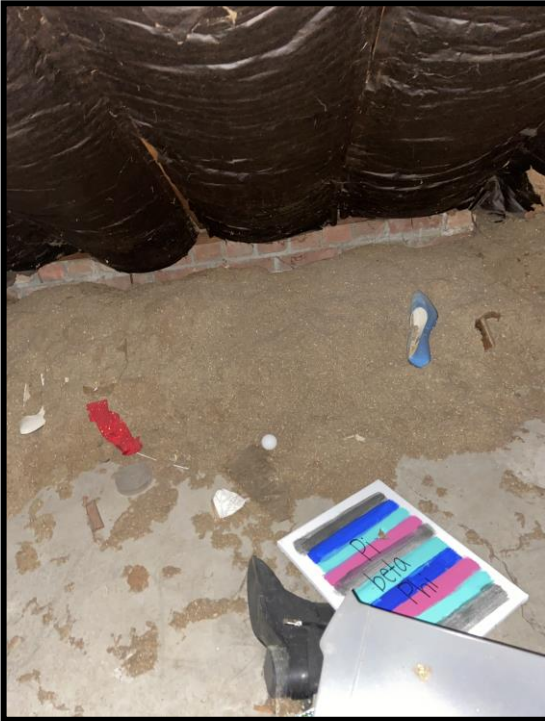
NON-ACM BLOWN-IN INSULATION IN ATTIC
