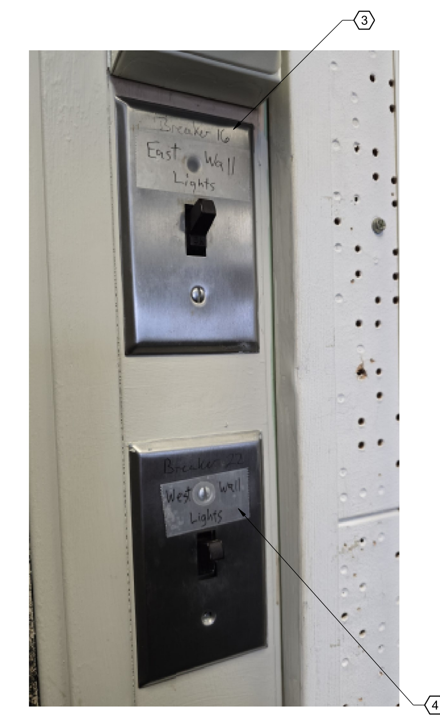
2 EXISTING SWITCH - PHOTO REFERENCE E002 NOT TO SCALE
