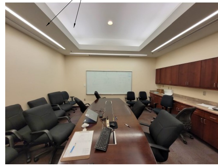
(E) GYP. BOARD CEILING AND SOFFIT TO BE REMOVED
