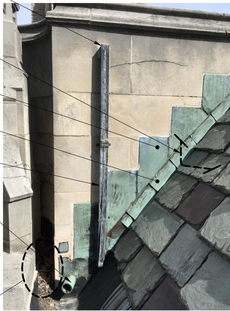
3 CENTER ROOF ELEVATIONS, TYP. N.T.S. NOTE: COUNTERFLASHINGS, GUTTER LINER DETAILS, AND SLATE BASE FLASHINGS SIM TO FR4.21 DETAILS FOR OPPOSITE END OF ROOFING.
