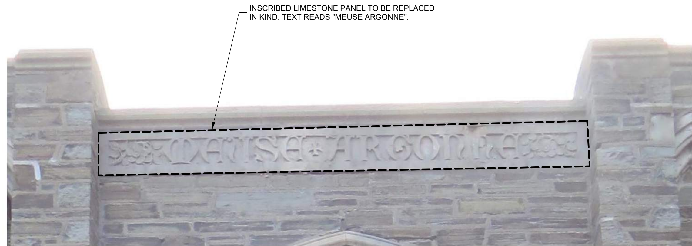
D DETAIL - TYPE D STONE REPLACEMENT (REFER TO DETAIL C/FR4.10 FOR ADDITIONAL INFORMATION)
