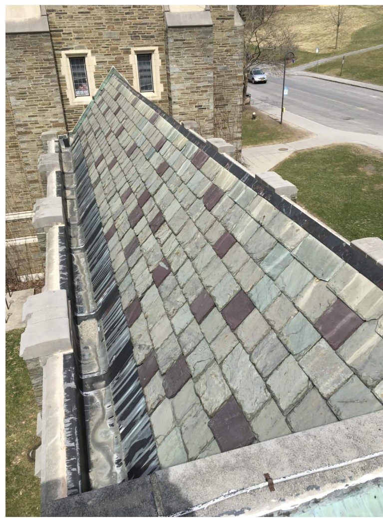
2 PURPLE SLATES LAYOUT, TYP. N.T.S. NOTE: PURPLE SLATES DISTRIBUTED RANDOMLY 3-4 SLATES PER COURSE.
