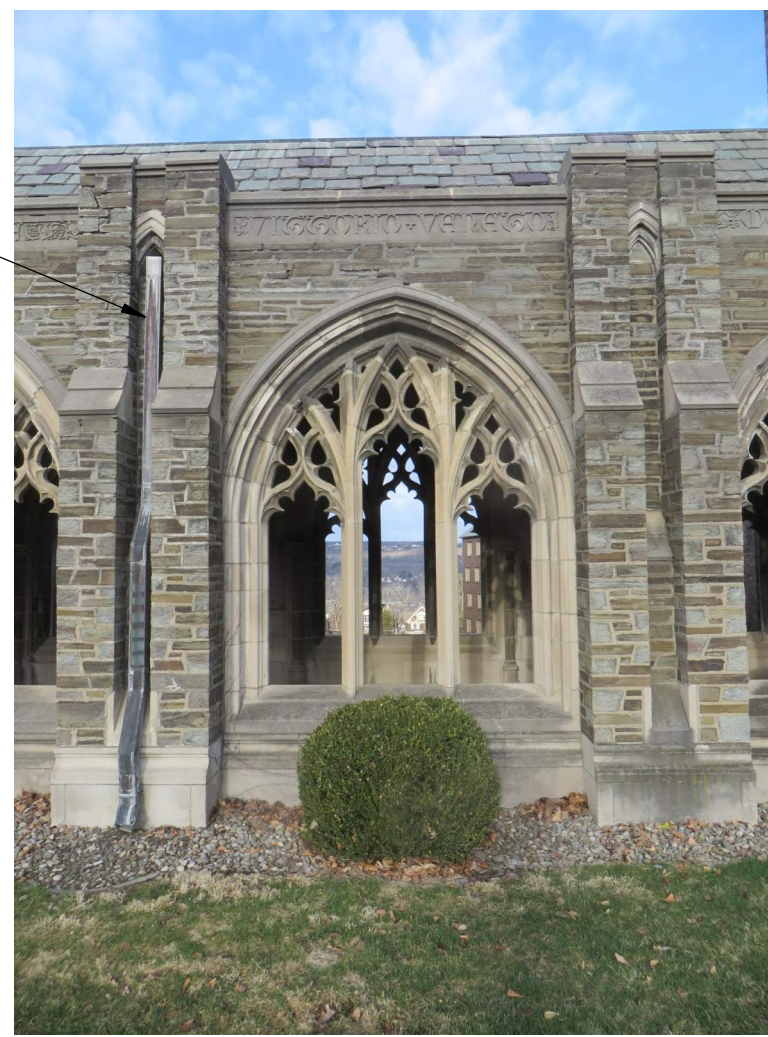
4 OVERVIEW - EXISTING DOWNSPOUT, TYP N.T.S. NOTE: REFER TO DETAIL 3/FR4.11 FOR INFORMATION ON MASONRY REPAIRS AT DOWNSPOUT REMOVAL LOCATIONS.
