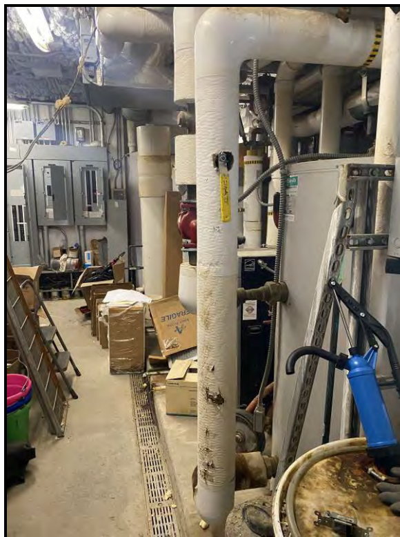
Non-Suspect Fiberglass Pipe insulation with Non-Asbestos End Cap Sealant
