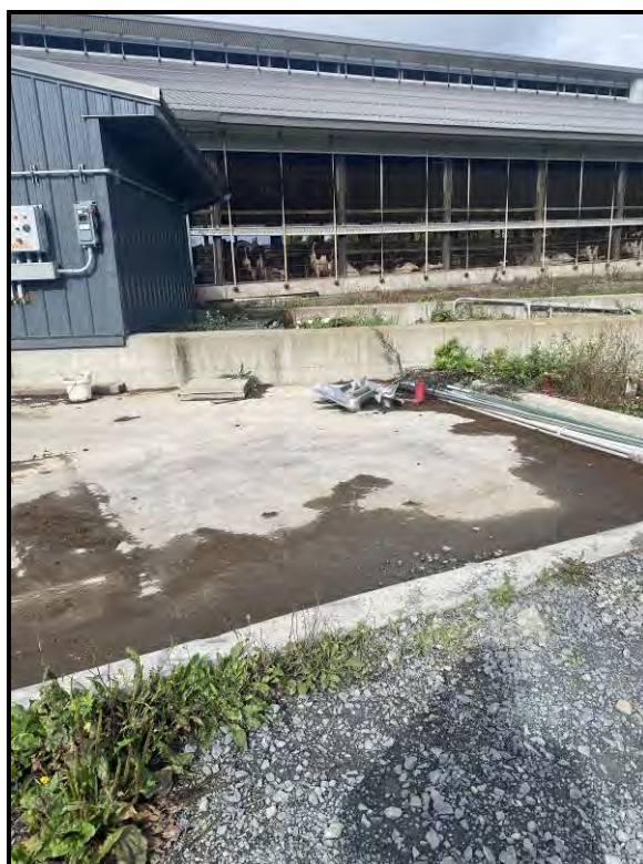
Exterior Surfaces with Non-Asbestos Joint / Seam Caulks
