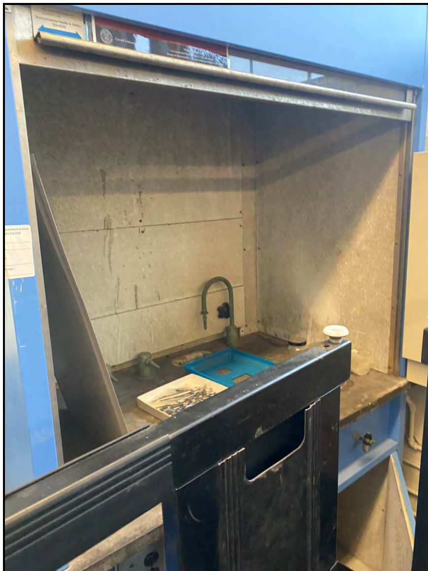
Room 309 asbestos transite lined fume hood / base cabinet and fume hood asbestos transite counter-top
