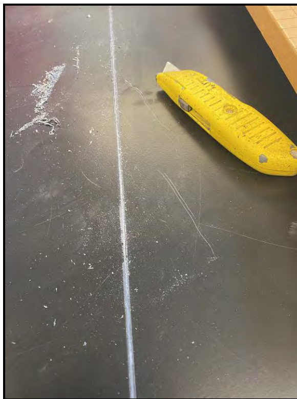
HA 03 – Counter-top Seam Epoxy, Room 309, “No Asbestos Detected”
