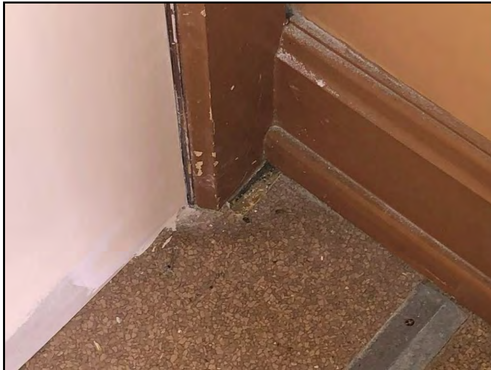
HA 01 – Brown Pebble-Pattern Linoleum, Corridor 100CA Area @ Rooms 105/107 Entry Area – “No Asbestos Detected”
