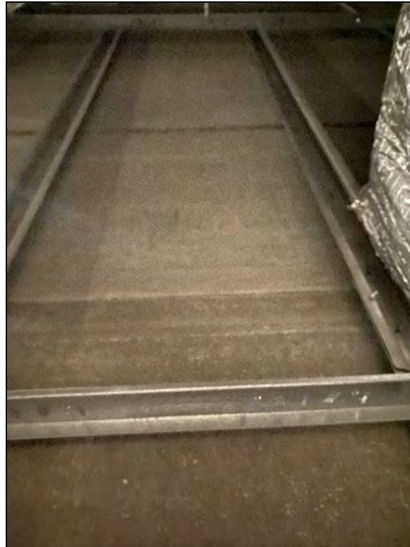
HA 03 – Cement Board Ceiling Panel, “No Asbestos Detected”
