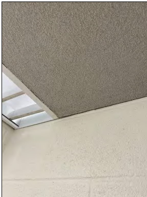
HA 06 – Textured Skim Coat, Ceiling, “No Asbestos Detected”
