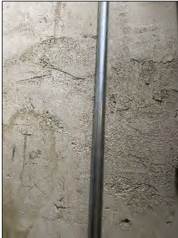
HA 13 – Wall Parging, “No Asbestos Detected”
