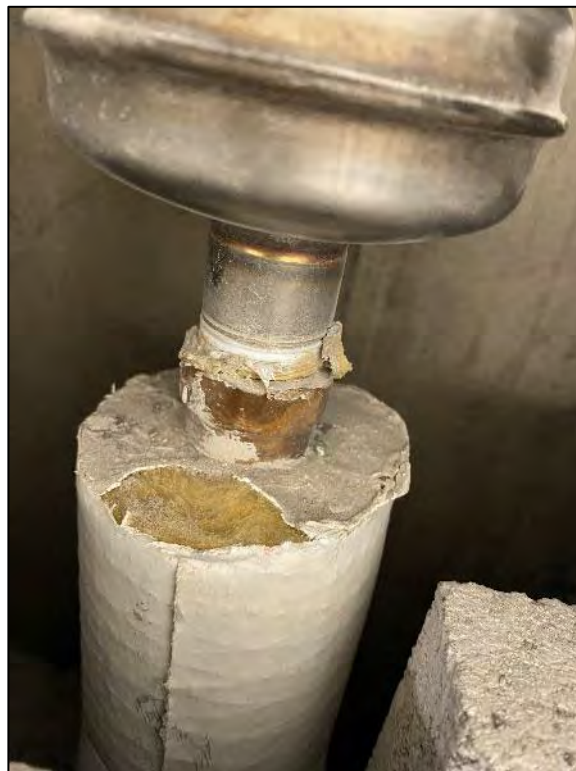
HA 04 – End Cap Sealant, “No Asbestos Detected”
