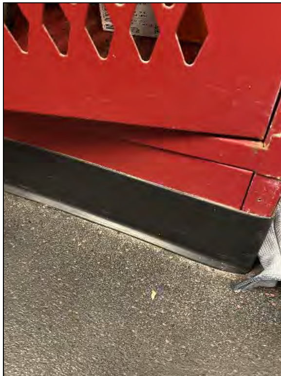
HA 10 – Mastic from 4” Non-Suspect Black Vinyl Cove Base, “No Asbestos Detected”
