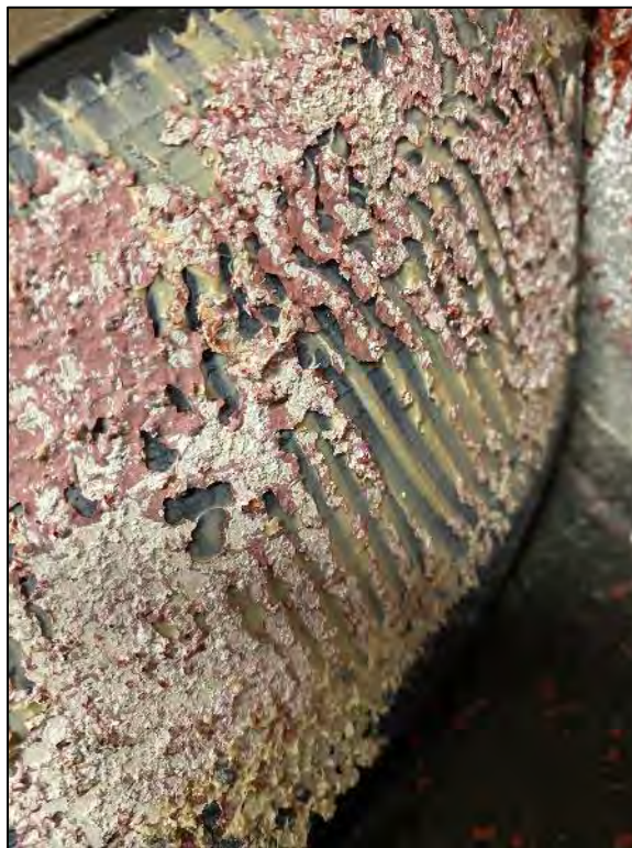
HA 02 – Mastic from 4” Non- Suspect Cove Base, “No Asbestos Detected”
