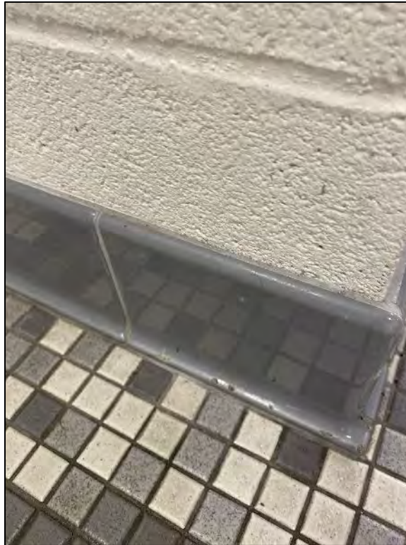
HA 05 – Grout/Mud Set from Grey 4” Ceramic Cove Base, “No Asbestos Detected”
