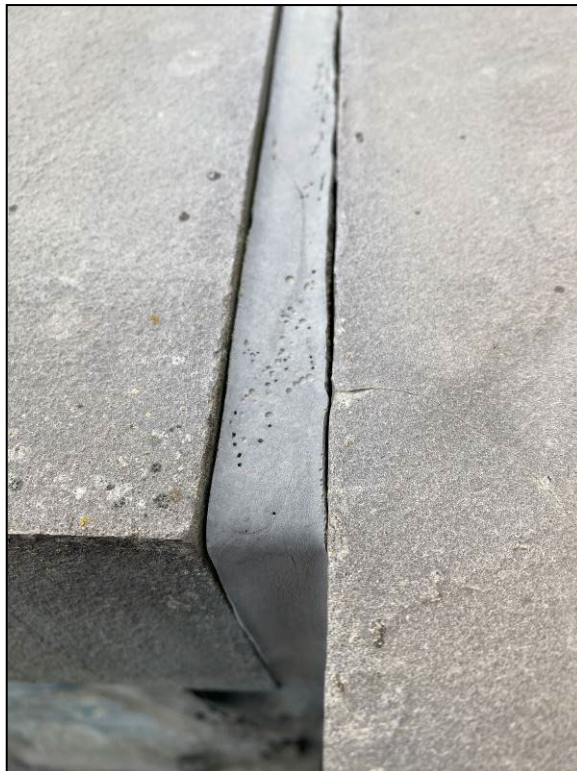
HA 02 – Grey Seam Caulk, Cap Stone, “No Asbestos Detected”
