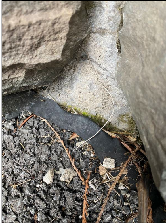
HA 03 – Black Caulk, Wall Base, “No Asbestos Detected”
