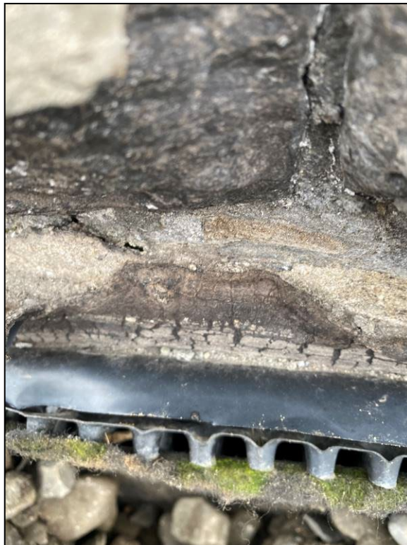
HA 06 – Foundation Waterproofing, “No Asbestos Detected”
