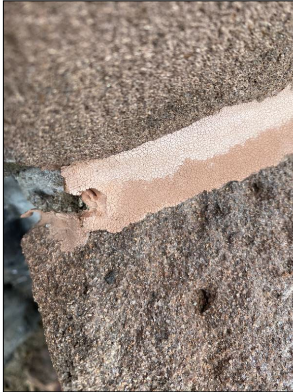
HA 01 – Caulk at Exterior Southwest Stairs, “No Asbestos detected”
