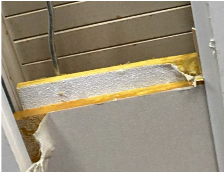
White Cloth Face from 2' x 8' Fiberglass Ceiling Tile, No Asbestos Detected Typical for HA's 09, 15 & 16
