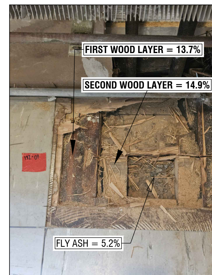
B SLM-101 VIEW OF MOISTURE READINGS, FLY ASH SAMPLE 132-01
