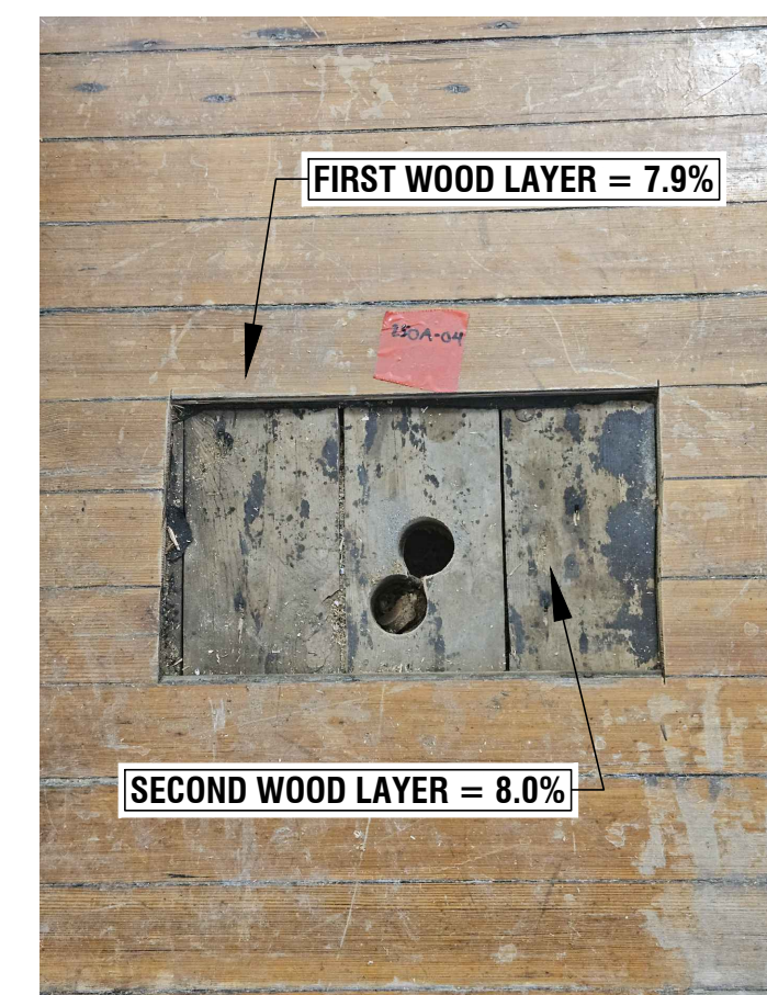
E SLM-101 VIEW OF MOISTURE READINGS, FLY ASH SAMPLE 250A-04
