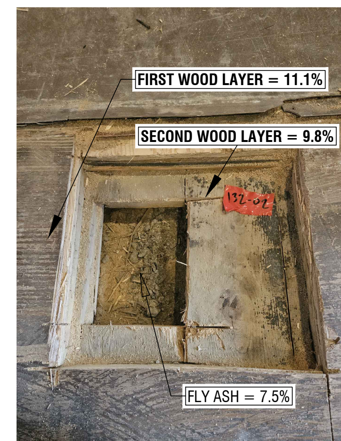
C SLM-101 VIEW OF MOISTURE READINGS, FLY ASH SAMPLE 132-02
