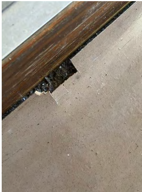
HA 14 - Brown Linoleum Sheet Flooring / Mastic Composite
