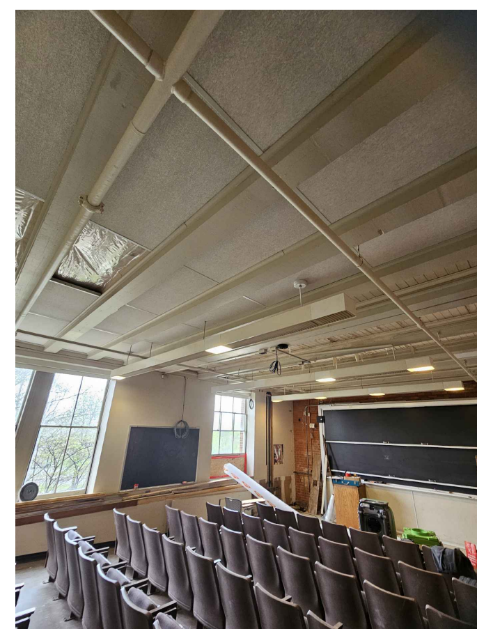
A CEILING GRID SYSTEM BETWEEN FLOOR JOISTS H-101
