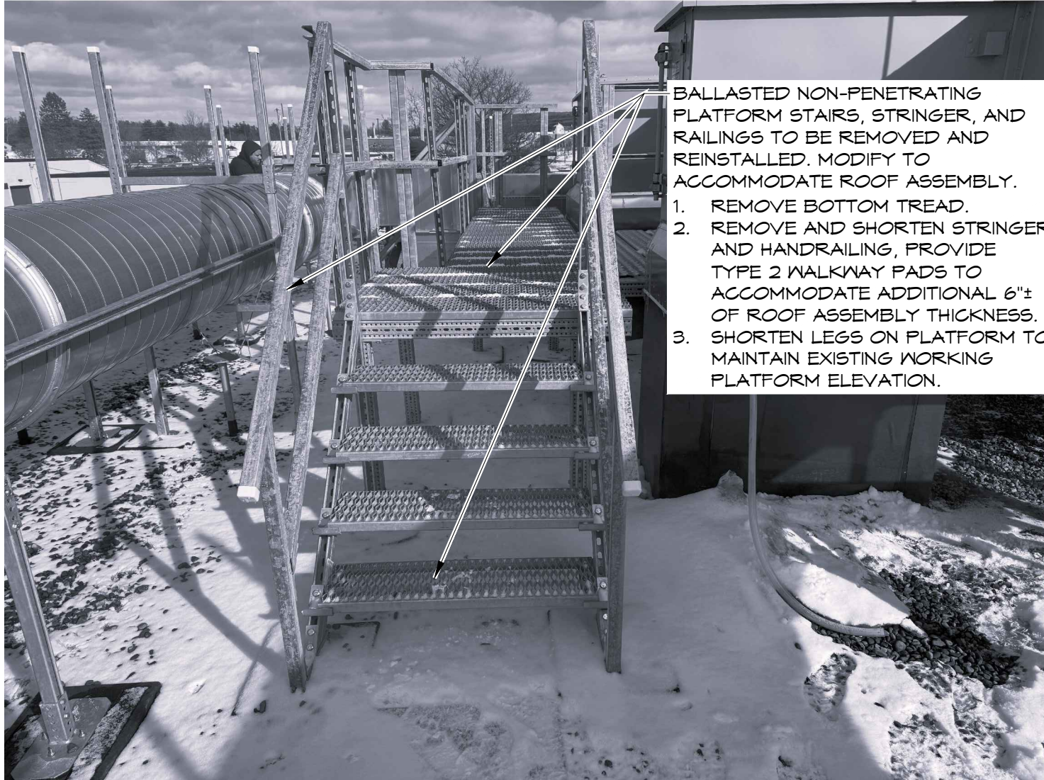
P11 - ROOF AREA 1164-001
