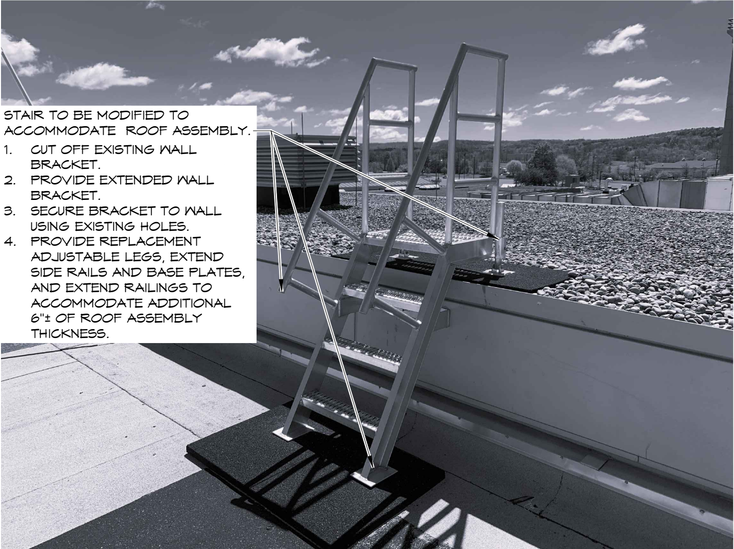
P12 - ROOF AREA 1164-001
