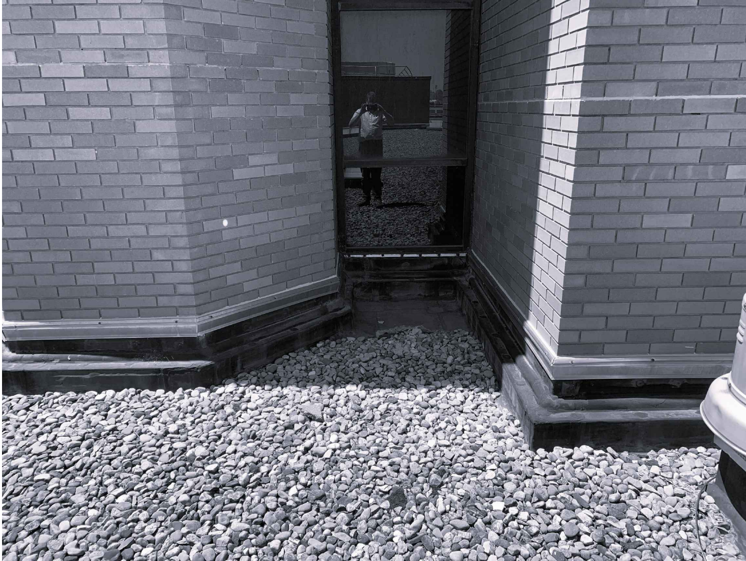
P2 - ROOF AREA 1163-001
