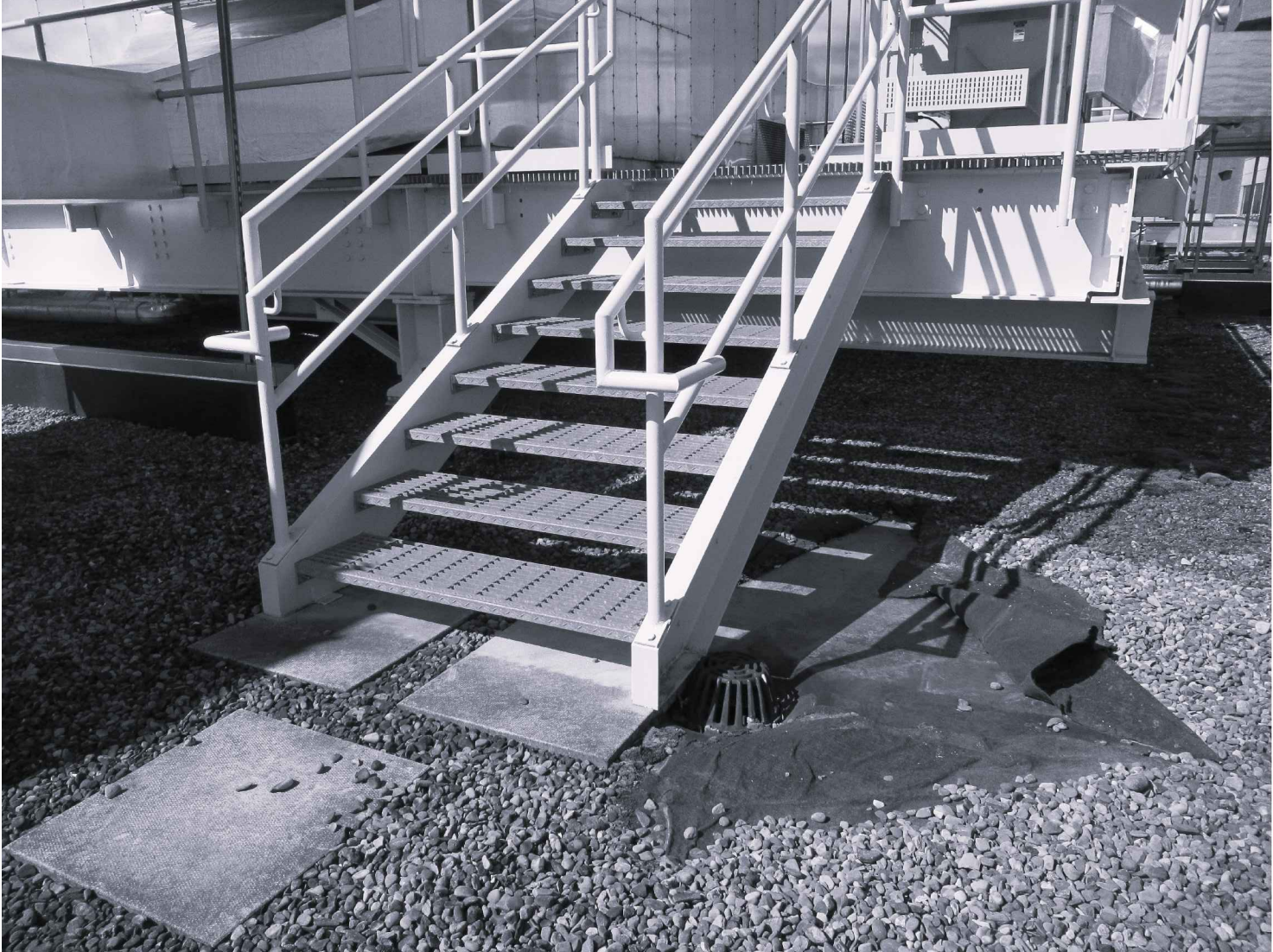
P4 - ROOF AREA 1164-001
