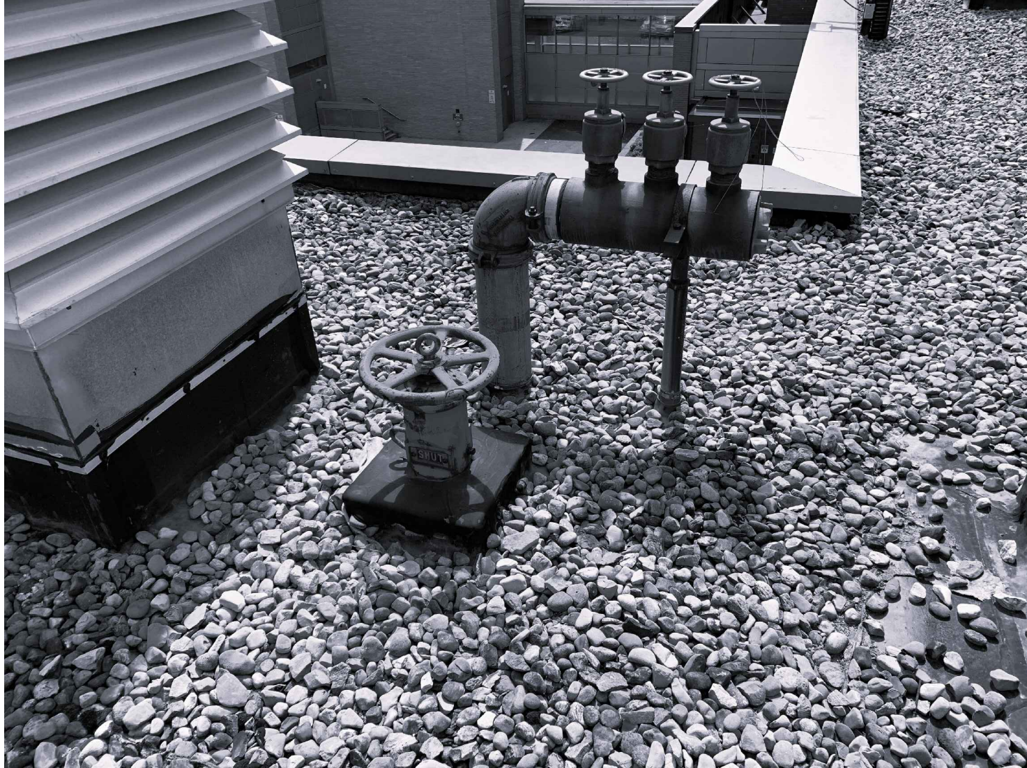
P1 - ROOF AREA 1163-001
