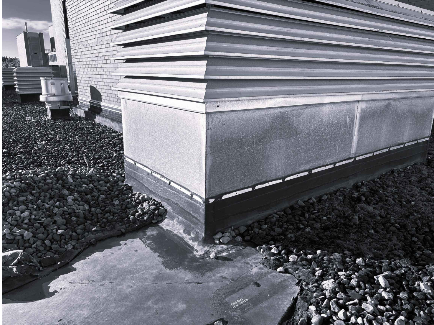
P3 - ROOF AREA 1163-001
