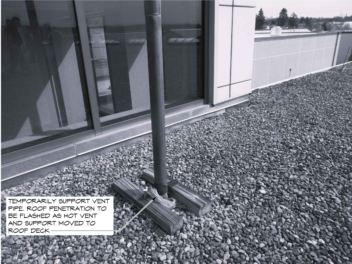
P10 - ROOF AREA 1164-001
