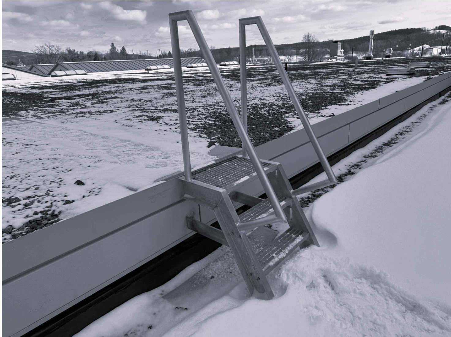
P7 - ROOF AREA 1164-007
