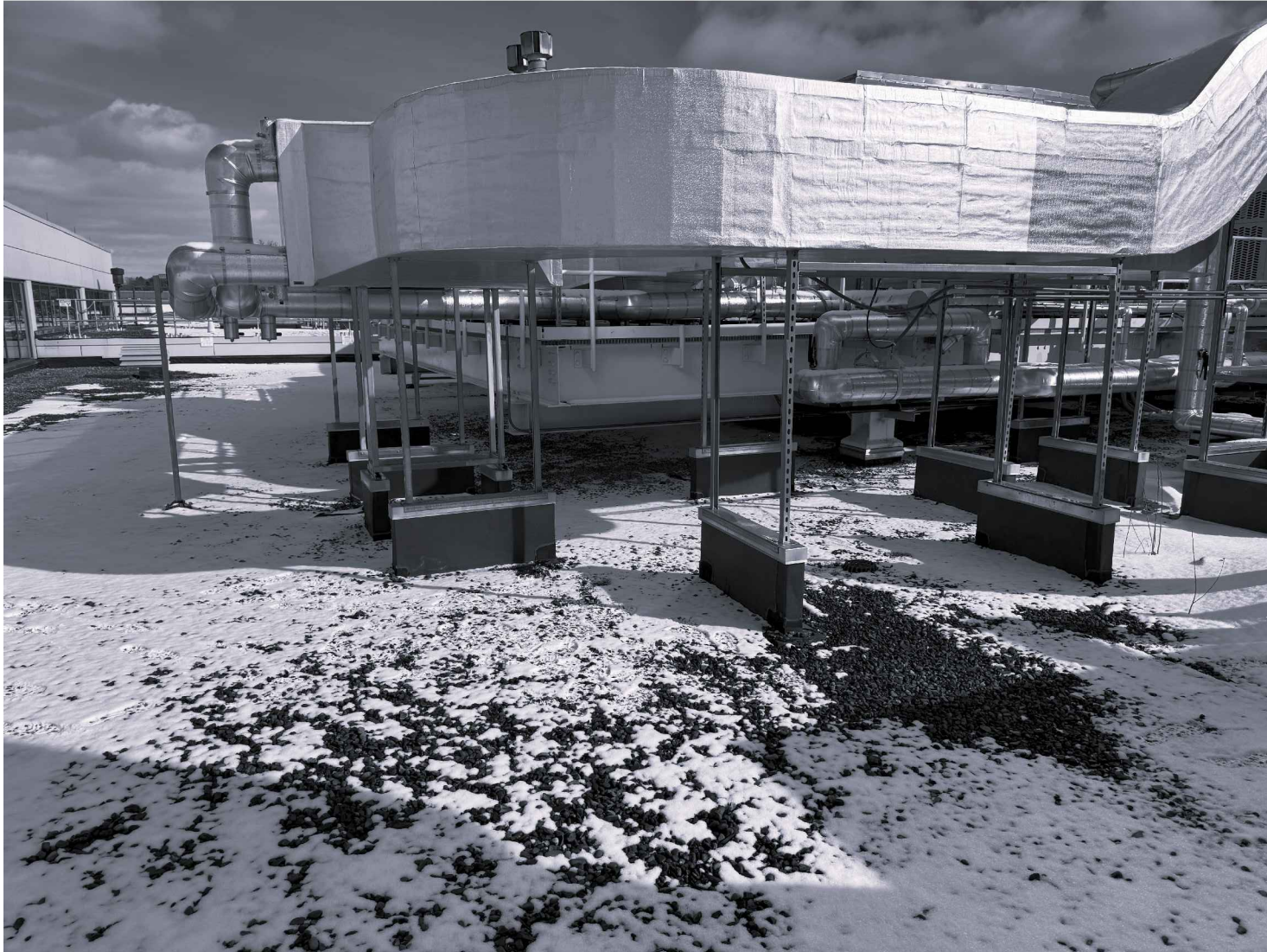
P6 - ROOF AREA 1164-001
