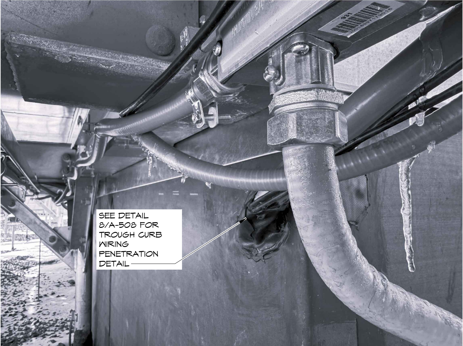
P8 - ROOF AREA 1164-007
