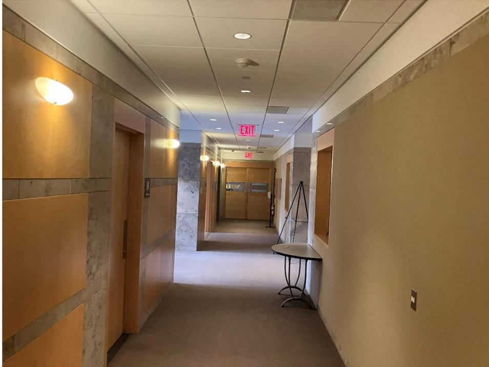
Photo 3: View of typical finishes on the 3<sup>rd</sup> floor. Wood and stone wall panels throughout the building are secured with clips and so are non-suspect for asbestos.
