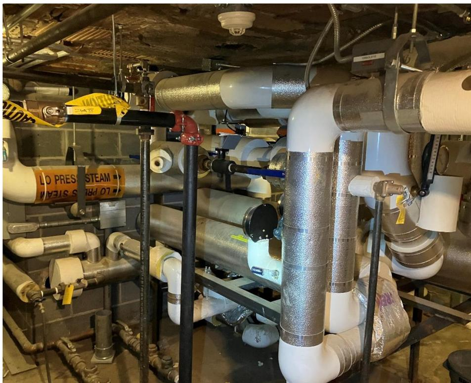
Photo 6: Typical view of mechanical piping in the building. All of the pipes and HVAC ducts that were observed above suspended ceilings were insulated with non-ACM fiberglass insulation.
