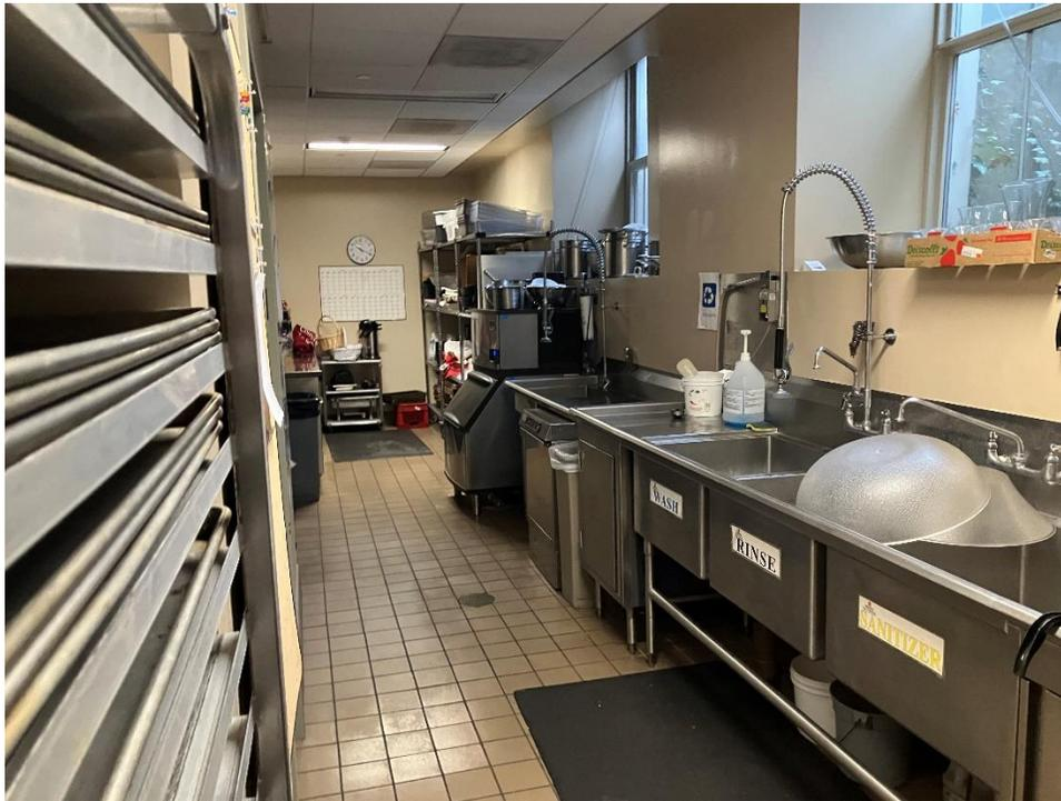
Photo 7: View of Kitchen 230. Quarry tile flooring and covebase grout and set were sampled and determined to be non-ACM.
