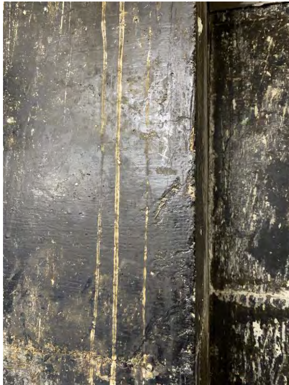
HA 10 - Tar Coating on Concrete Walls, No Asbestos Detected
