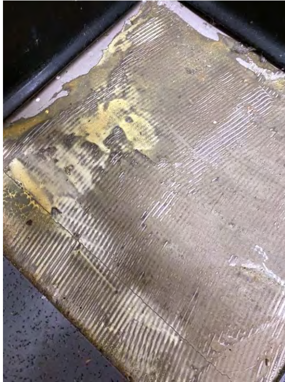
HA 07 - Mastic from Gray 12" x 12" Floor Tile, No Asbestos Detected
