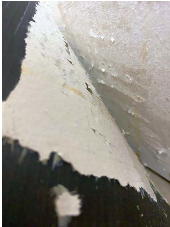
HA 08 - Mastic from non-suspect 6" Vinyl Cove Base, No Asbestos Detected
