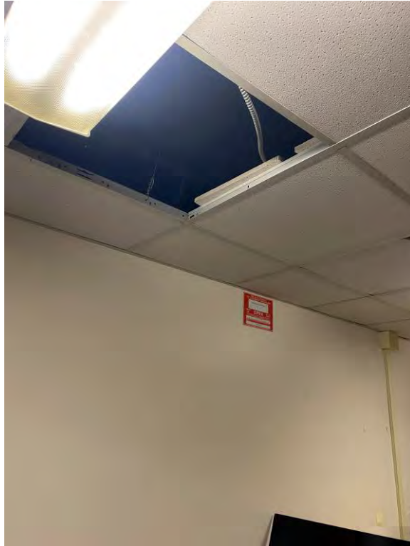
HA 09 - 2' x 2' Hole-Pattern Ceiling Tile, No Asbestos Detected
