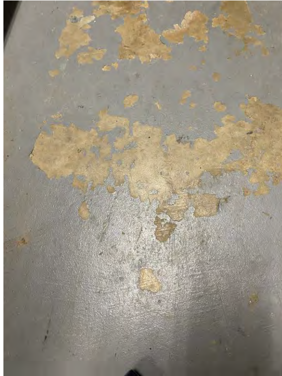
HA 11 - Gray Epoxy Flooring, No Asbestos Detected
