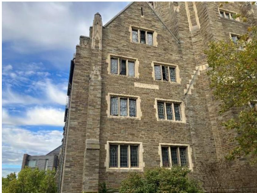
Photo 1: View of McFaddin Hall. Mortar associated with the buttress was sampled as part of this investigation and was determined to be non-ACM.
