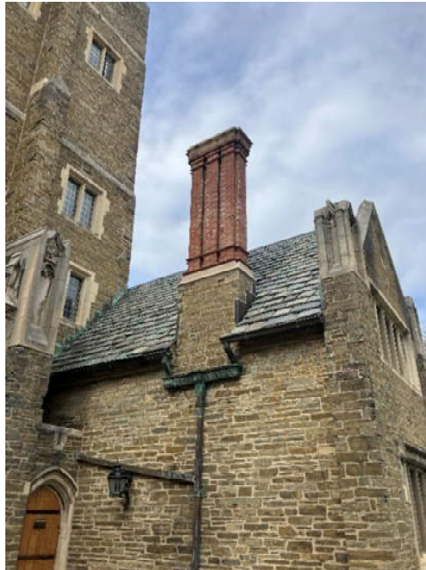
Photo 2: View of a typical chimney at the Gothics Complex that is scheduled to be removed down to the roof level. Chimneys were not accessible for sampling during the inspection and will have to be inspected during construction for suspect asbestos-containing materials.
