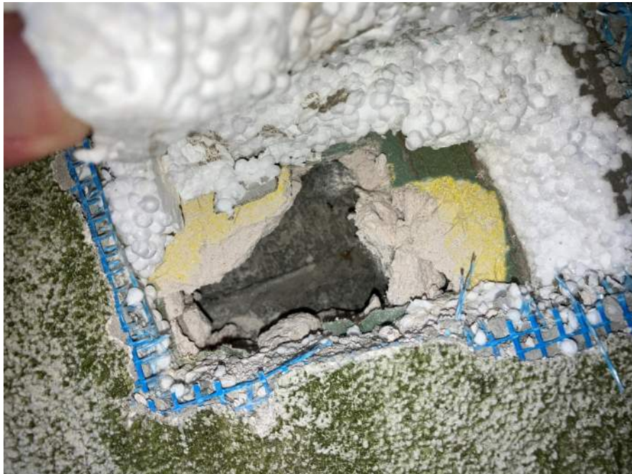
Photo 4: Close up view of the EIFS. All suspect materials anticipated to be impacted by the project were determined to be non-ACM.
