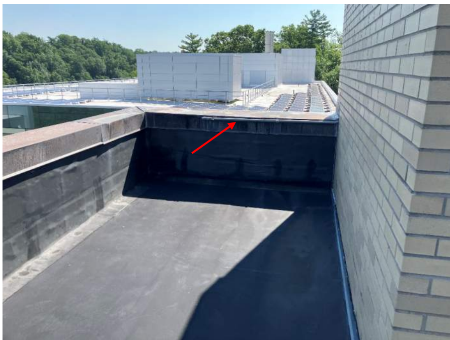
Photo 2: View of the section of the upper roof scheduled to be impacted as part of the project. Gray caulk at the metal coping and firestop caulk at the conduit (arrow) were determined to be non-ACM.
