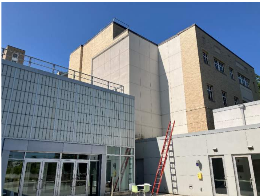
Photo 1: View of MVR West and the EIFS panels that are to be replaced as part of the project.
