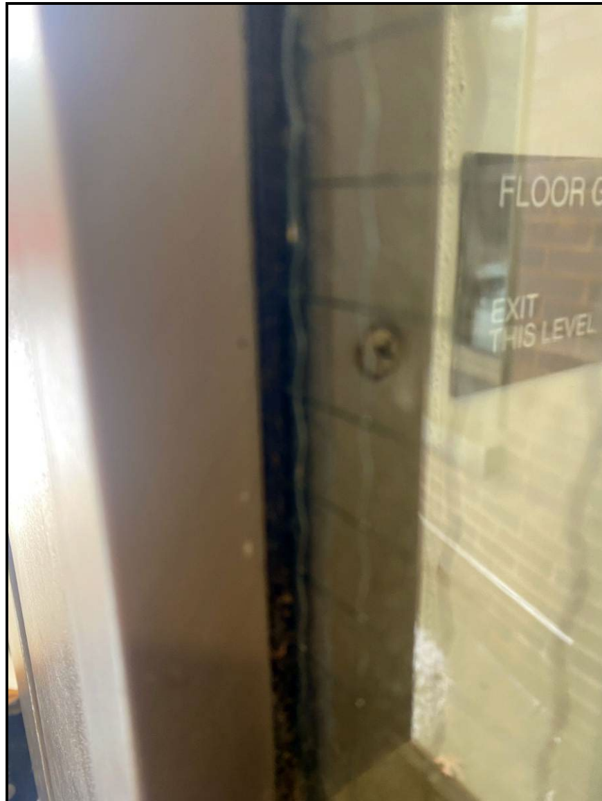
HA 01 – Stairwell G0001 Exterior Entry Door Window Glazing Compound Non-Asbestos” (< 1.0%)
