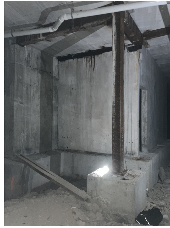
9 INTERIOR WORK AREA VIEW 2 PHOTO REFERENCE
