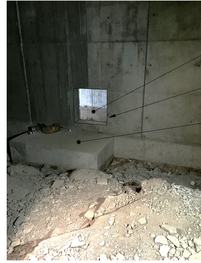
7 INNER OPENING AS SEEN FROM BASEMENT WORK AREA PHOTO REFERENCE
