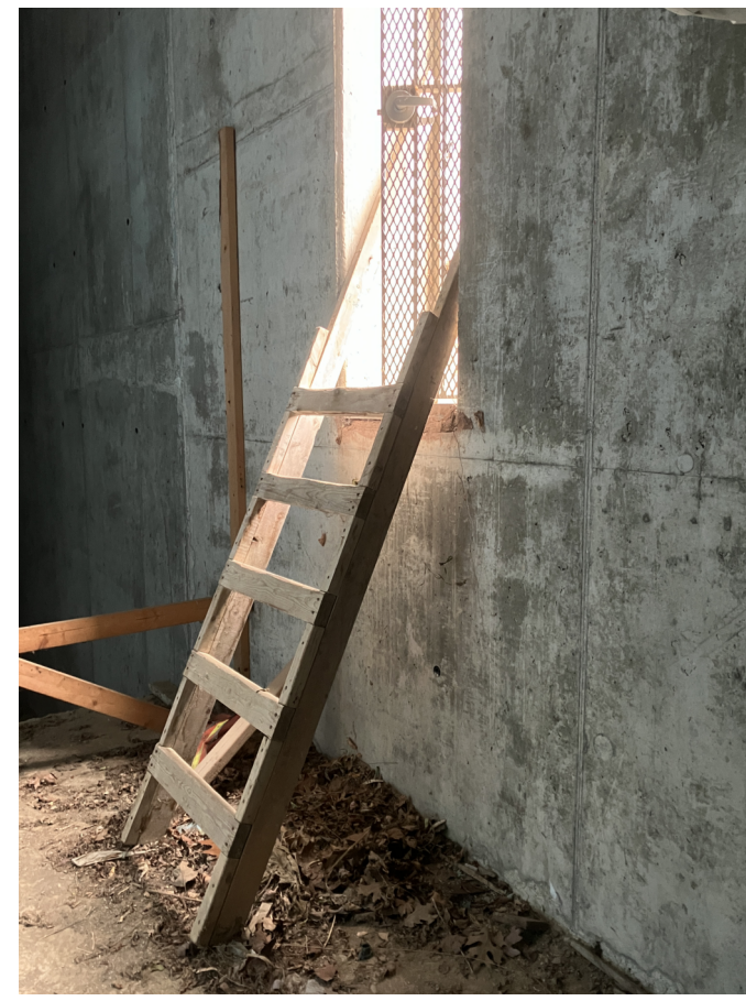
6 INSIDE VIEW OF LOUVER PHOTO REFERENCE
