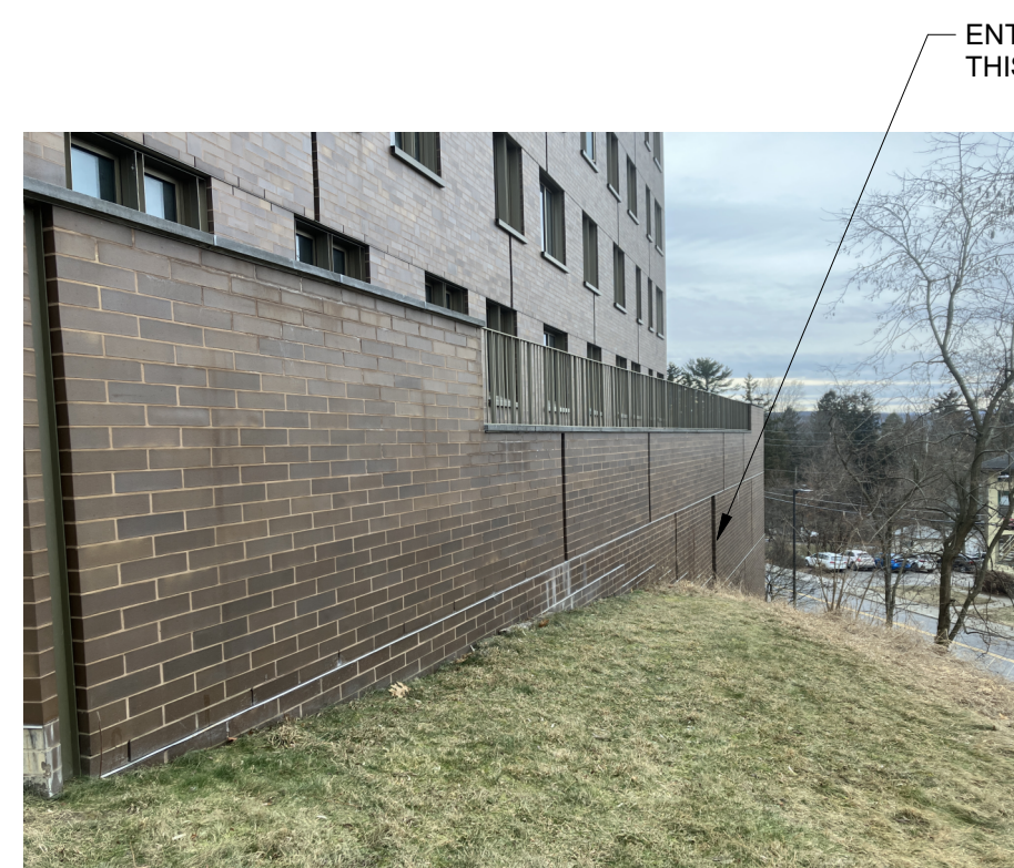
4 EXTERIOR VIEW PHOTO REFERENCE
