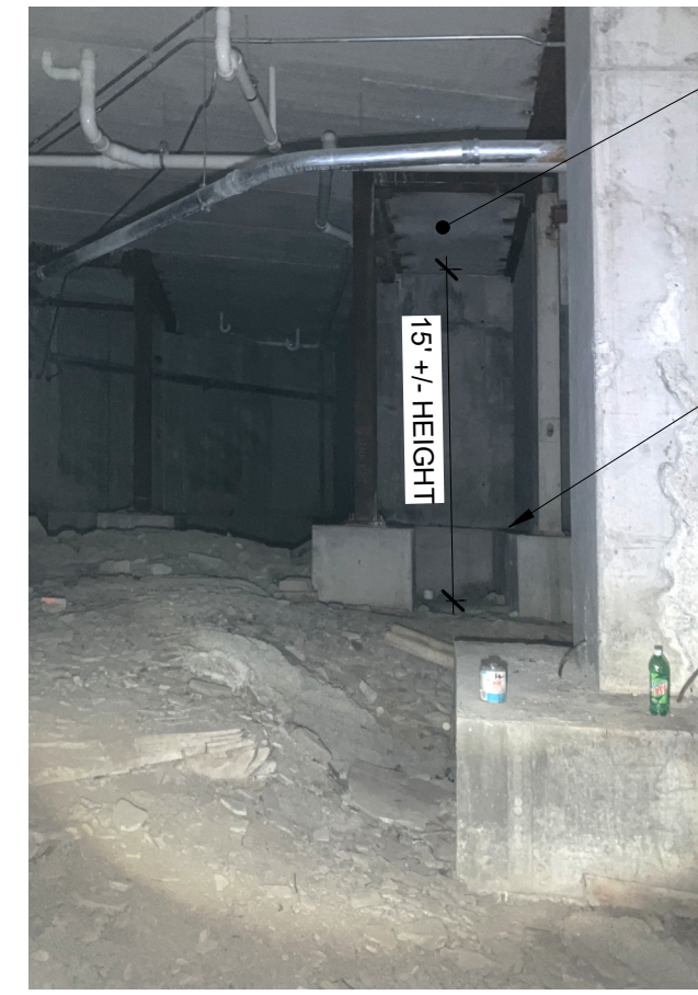
8 INTERIOR WORK AREA VIEW 1 PHOTO REFERENCE
