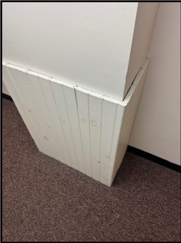
WOOD WASN'T REMOVED TO SEE IF THERE WAS MASTIC, WOULD NEED TO BE CHECKED BEFORE DEMOLITION OF THE WOOD
