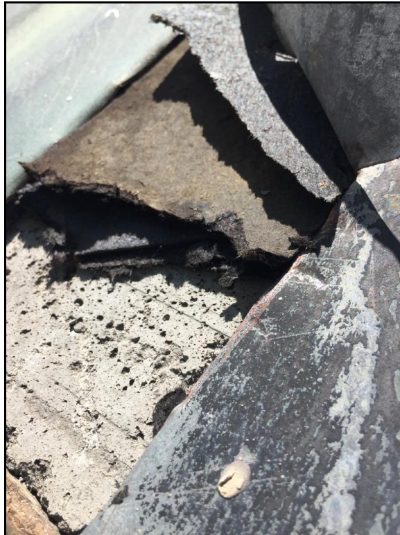
HA 03 – Vapor Barrier on Concrete, “No Asbestos Detected”
