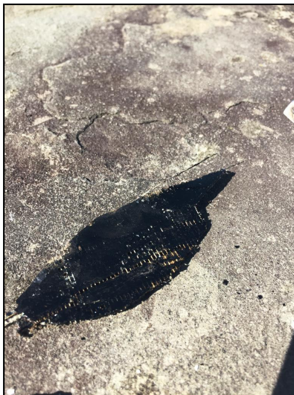
HA 10 – Chimney Flue Repair Fabric, “No Asbestos Detected”
