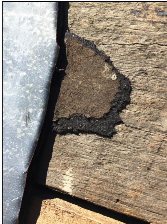
HA 02 – Vapor Barrier on Wood Below Dormer, “No Asbestos Detected”
