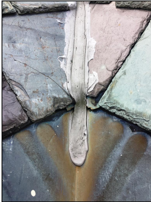
HA 07 – Valley Repair Caulk, “No Asbestos Detected”
