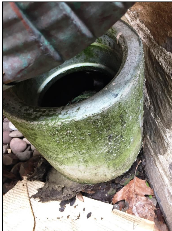
HA 12 – Rain Water Conductor Transite Drainage Pipe, “Asbestos Containing”
