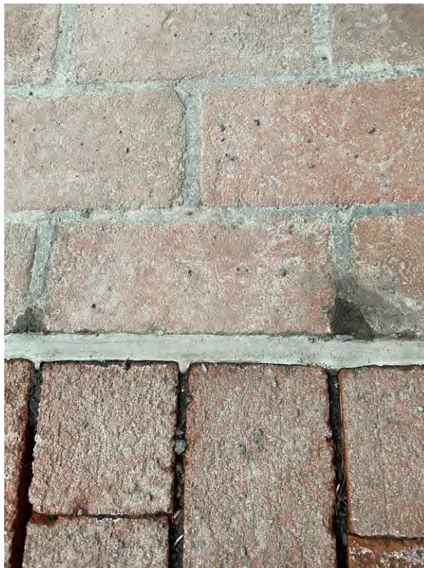
HA 02 – Grey Seam Sealant, Front Entrance Ramp, “No Asbestos Detected”
