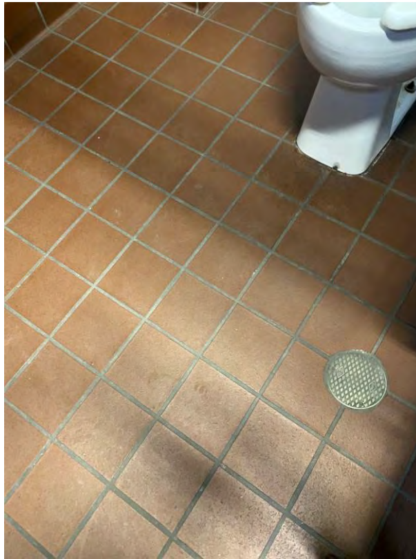
HA 01 – Grout / Mudset from non-suspect quarry tile flooring, “No Asbestos Detected”
